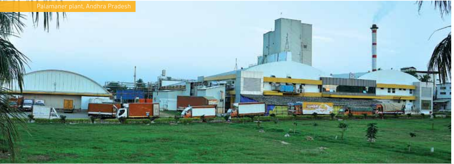
UHT facility at Palamaner plant
