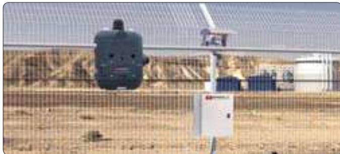
RoboGuard is a revolutionary agile scout robot, which runs along secured fences, ensuring perimeter integrity and capable of responding promptly to intrusion alerts. It consists of an autonomous unit, travelling on a monorail and carrying several sensors. (photo credits: magal)
