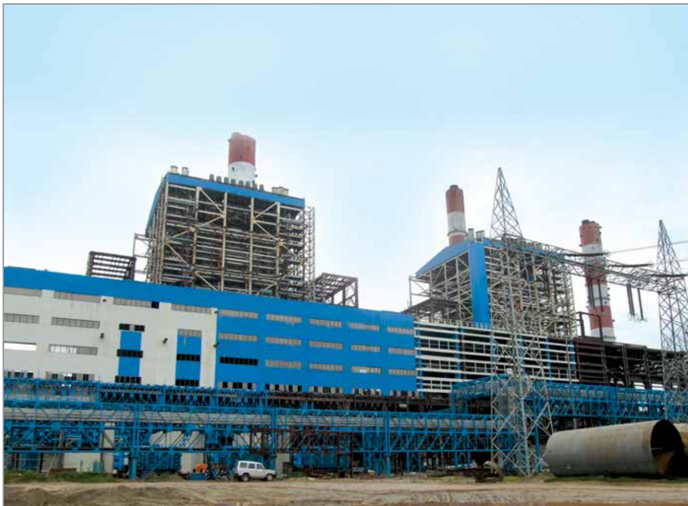
2x660 MW Barh Supercritical Power Project under execution by BHEL
