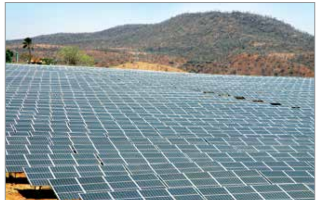
Grid-connected 5 MW Solar PV plant in Karnataka
