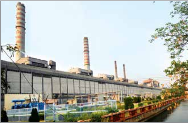
BHEL-built 200 MW (Unit 5) Singrauli STPS clocked uninterrupted operation throughout the year
