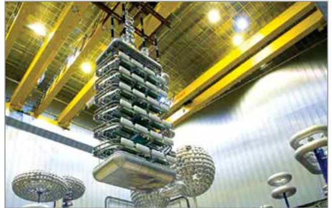
Thyristor Valve modules under Di-electric testing for \pm 800 kV, 6000 MW NE-Agra HVDC Project
