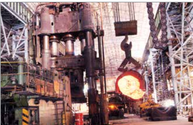
500/600 MW Rotor forging facility at CFFP, Haridwar
