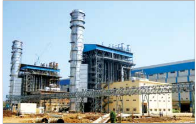
2x363 MW Gas-based Power Plant, OTPC-Palatana
