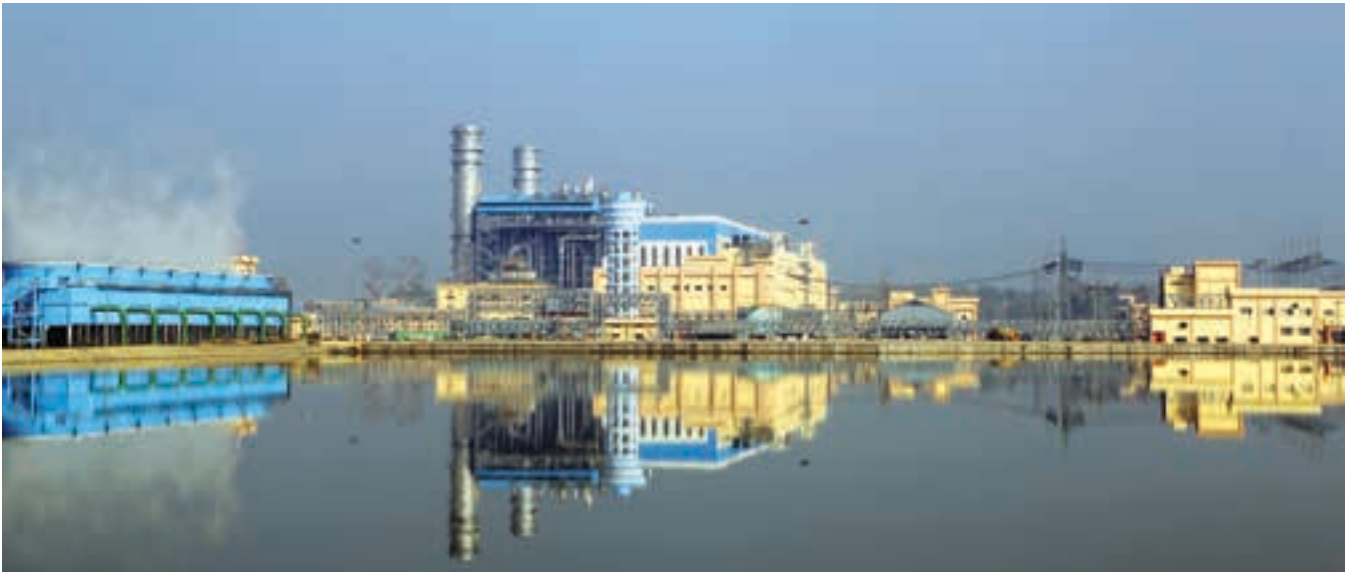
2x363 MW Gas-based Power Plant, OTPC-Palatana
