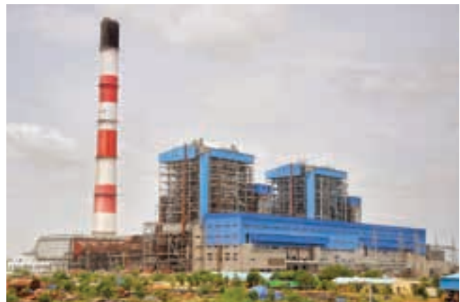
India's first indigenously manufactured 800 MW Boiler synchronised at Krishnapatnam
