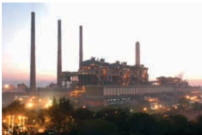
Korba STPS with BHEL supplied equipment recorded PLF more than 90%
