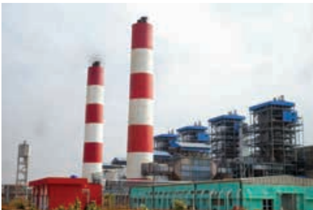
4x125 MW Unit 3 & 4, Kosti Thermal Power Plant executed in Sudan
