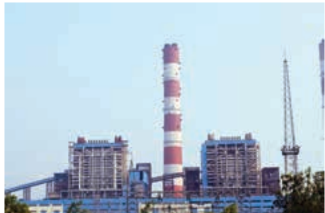
BHEL's first super-critical set of 660 MW rating commissioned at NTPC Barh Stage-II
