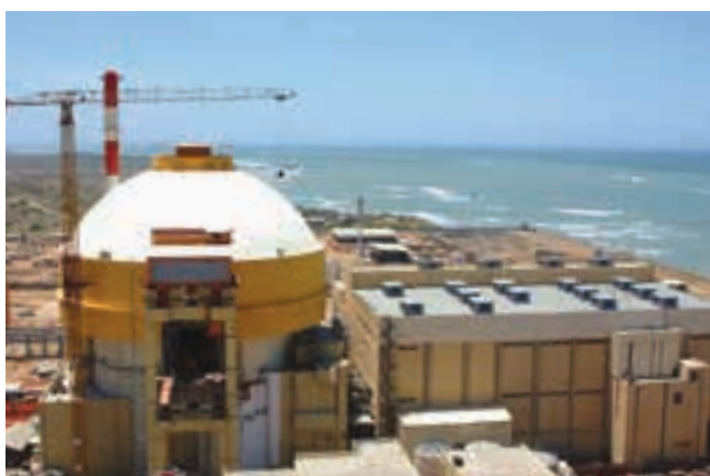
India's first 1000 MW Nuclear set at Kudankulam-1 synchronised by BHEL
