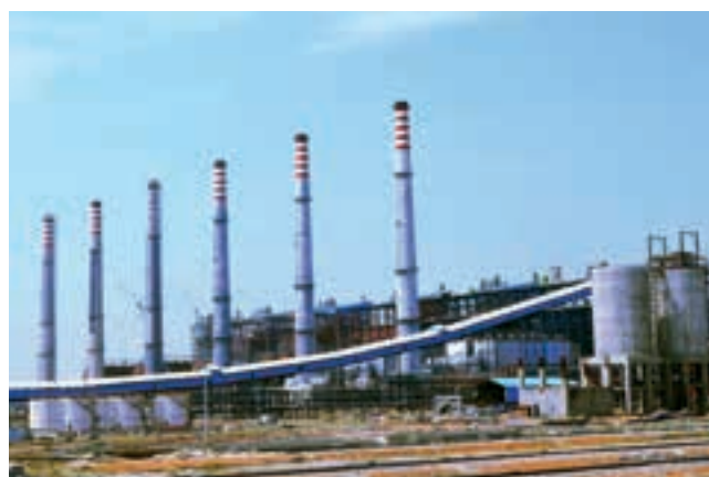
Unit – 2 & 3 of HINDALCO Industries Ltd. - Mahan Aluminium (300 MW) commissioned by BHEL
