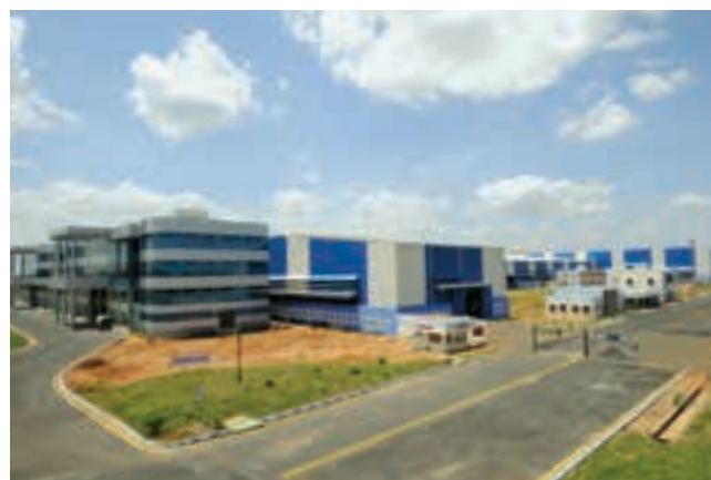
‘Power Plant Piping Unit’ established at Thirumayam, to manufacture High Pressure & Critical Piping for power plant applications
