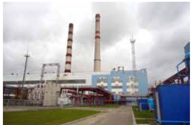
126 MW Grodno-II, Gas Turbine based Cogeneration Power Plant executed in Belarus
