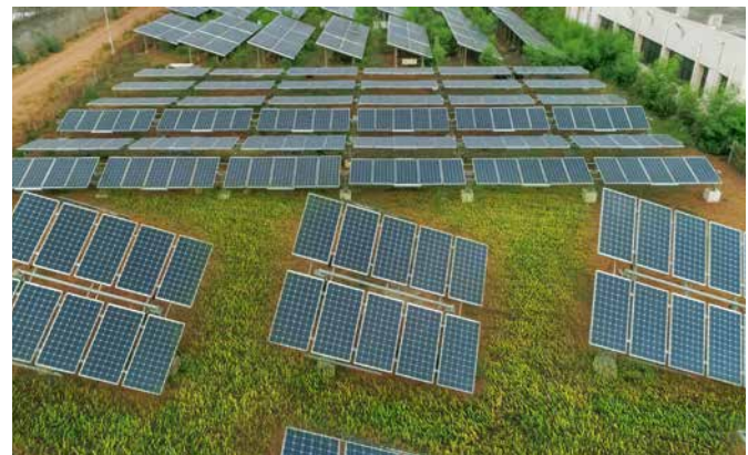
In-house solar installation at Corporate R&D, BHEL Hyderabad
