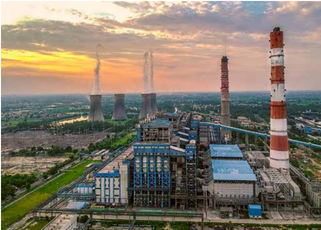
BHEL make FGD will be commissioned at older thermal units such as NTPC Dadri
