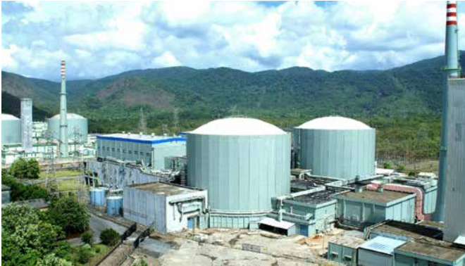
NPCIL Kaiga equipped with BHEL manufactured Turbine-Generator sets
