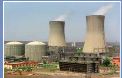
Rajasthan Atomic Power Station (RAPS) equipped with BHEL supplied Nuclear Steam Generators
