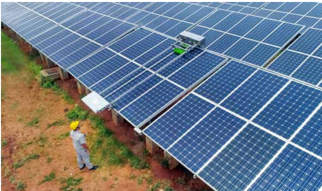
Indigenously developed solar cleaning panel robot under operation at BHEL Corporate R&D, Hyderabad
