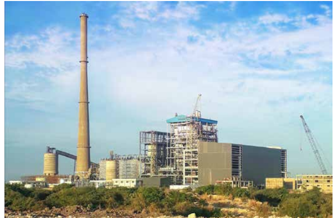
1x125 MW Sendou Thermal Power Project, Senegal
