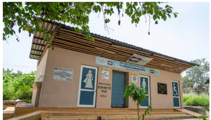
Bio-digester toilets on the banks of river Ganga near Haridwar & Rishikesh, installed by BHEL
