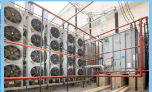
1200 KV Bina Sub-station equipped with BHEL supplied Transformers
