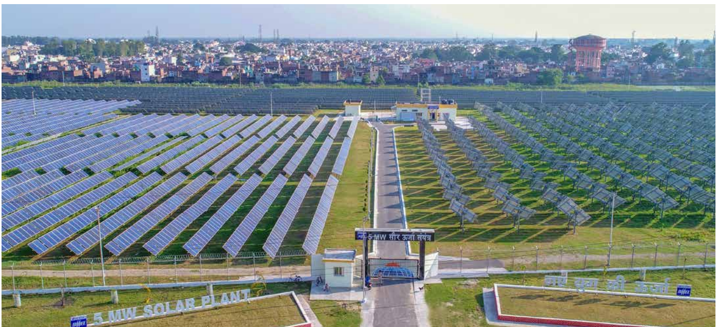
5 MW Solar Power Plant including ground mounted fixed, motor tracking and passive tracking enabled modules of BHEL make at Haridwar plant premises
