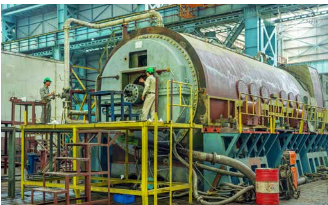
800 MW Generator testing at BHEL's Haridwar plant
