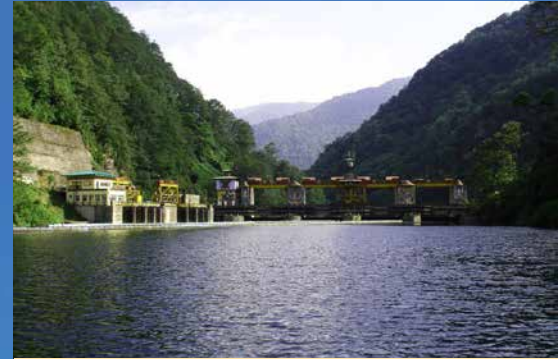
336 MW Chhukha HEP project executed by BHEL
