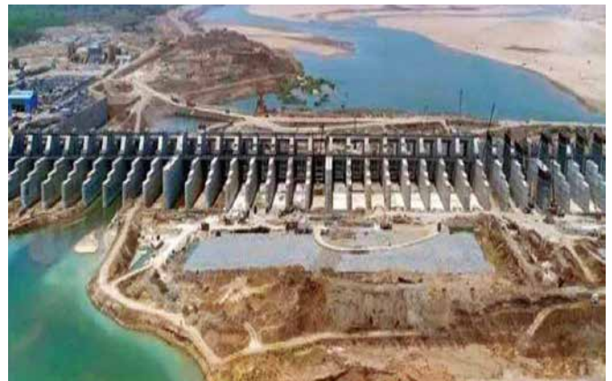
Kaleshwaram Lift Irrigation Scheme equipped with largest rating vertical pump-motor sets along with associated auxiliaries
