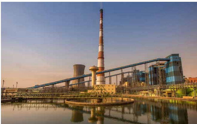
Clarifloculator at Bellary TPS. BHEL provides a complete range of water related solutions for power plants.
