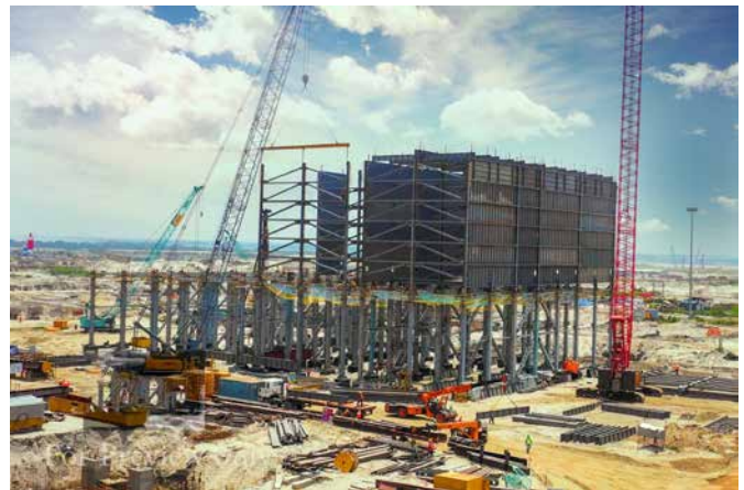
Erection work in progress at 2x660 MW Maitree project in Bangladesh
