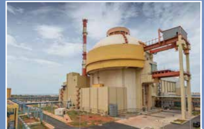
BHEL setting up NPCIL's Kudankulam Nuclear Power Project Units 3 & 4
