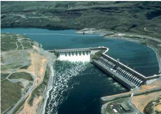
BHEL aided restoration, synchronisation to grid and operationalisation of Generating Unit 1 of the 336 MW Chhukha Hydropower Plant, Bhutan
