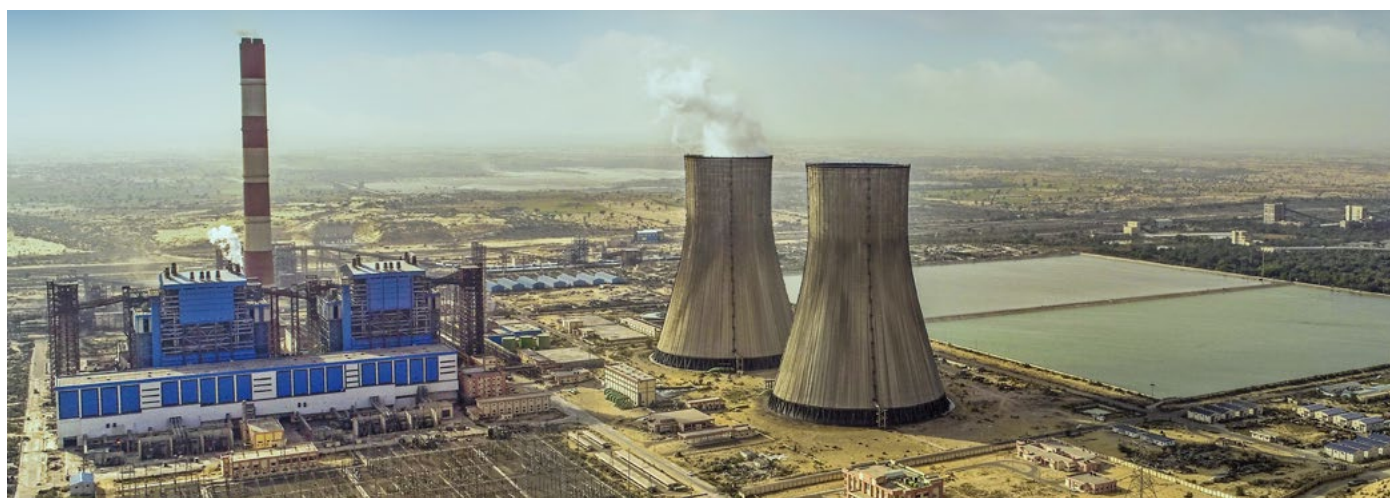
2x660 MW Super critical power plant under commissioning by BHEL at Suratgarh, Rajasthan
