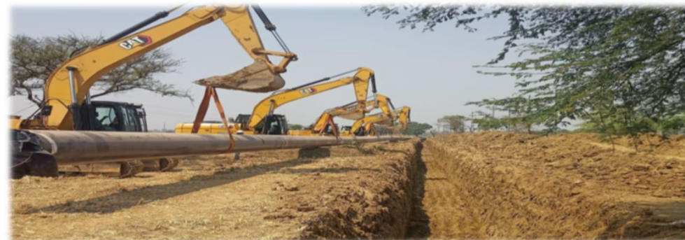
Setting up slurry pipeline
