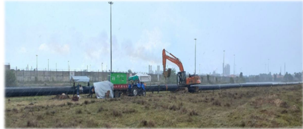
Setting up slurry pipeline
