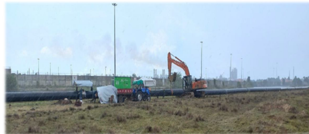
Setting up slurry pipeline
