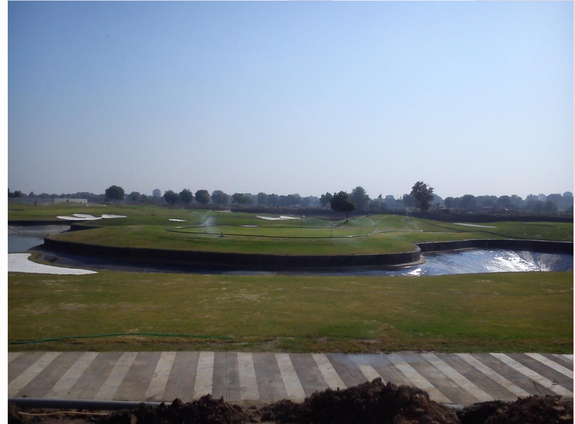
Golf Course Construction
