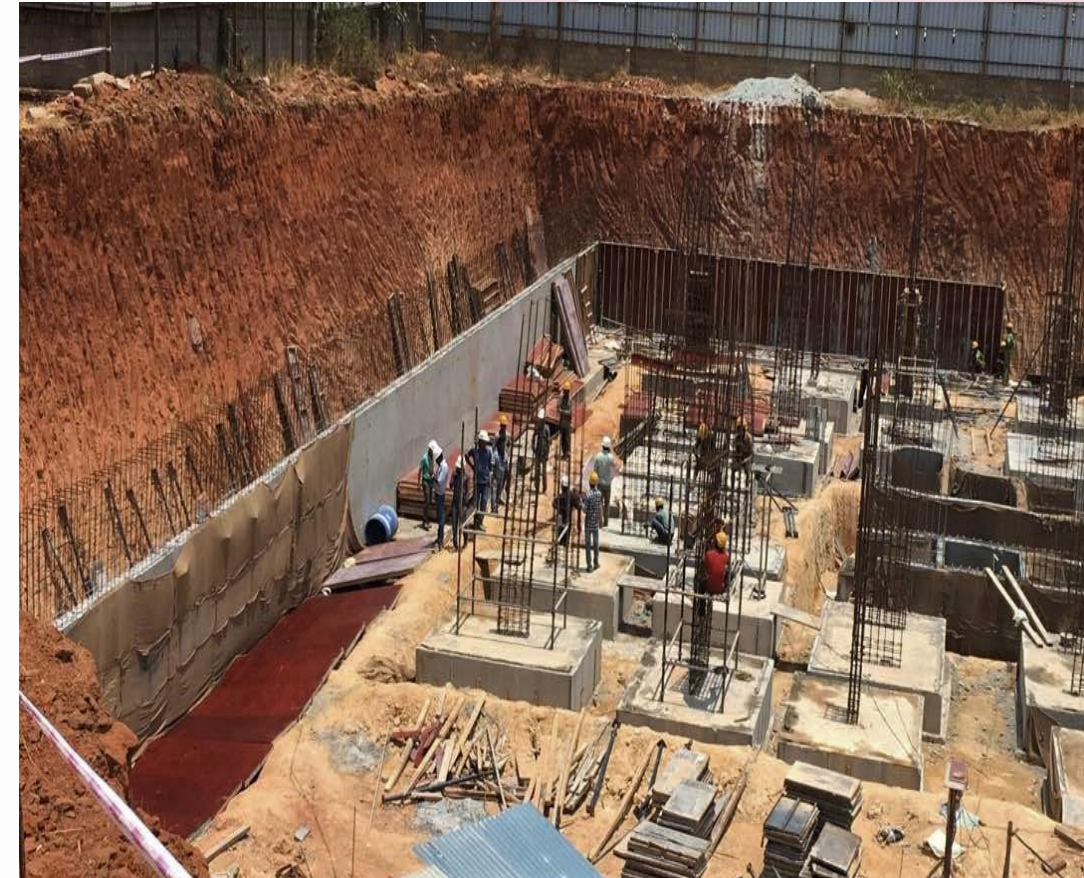
Retaining Wall Work at Site
