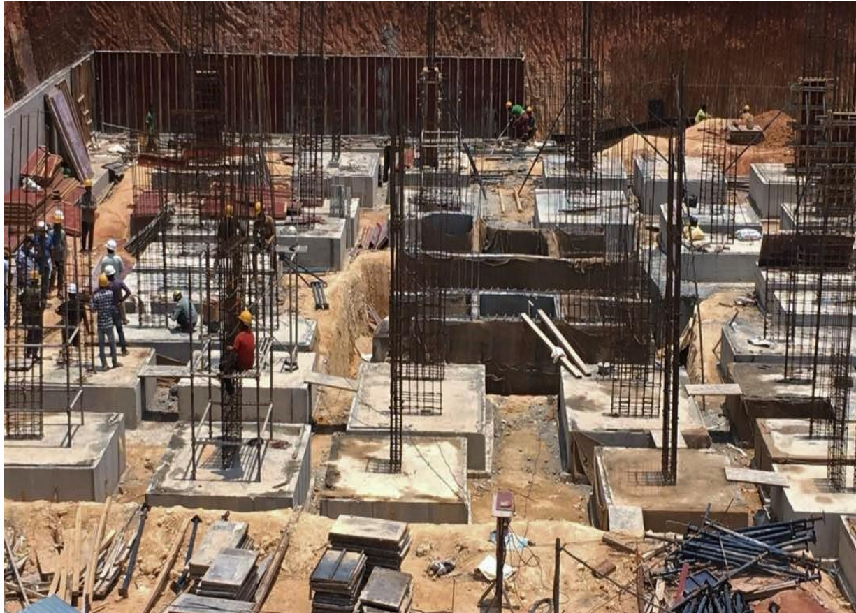
Foundation Work at Site
