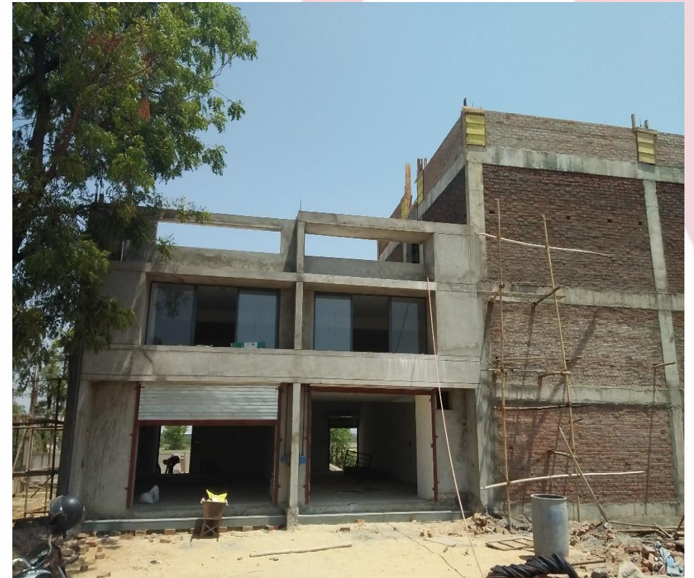
Construction work at Site
