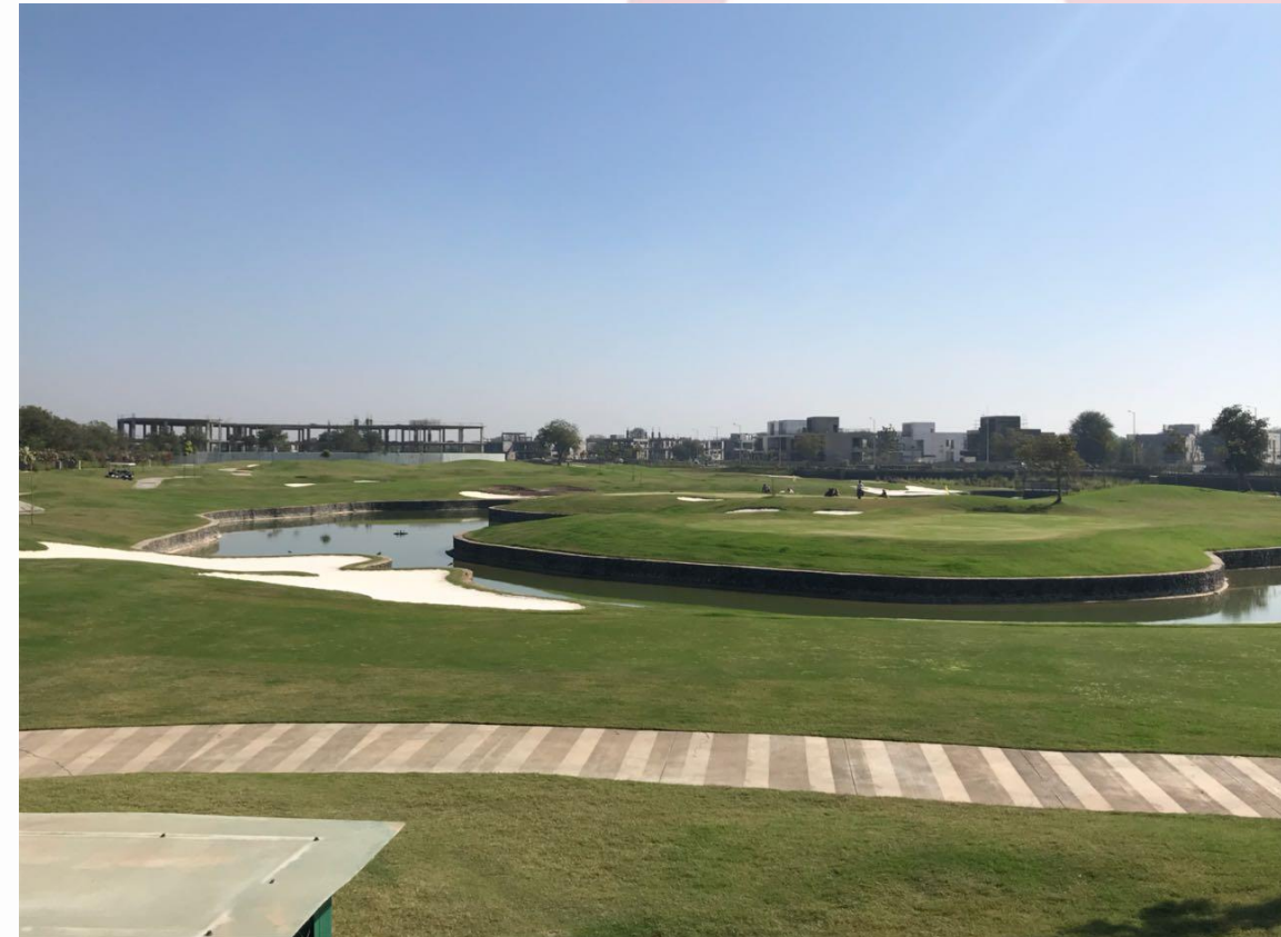
Golf Course Construction
