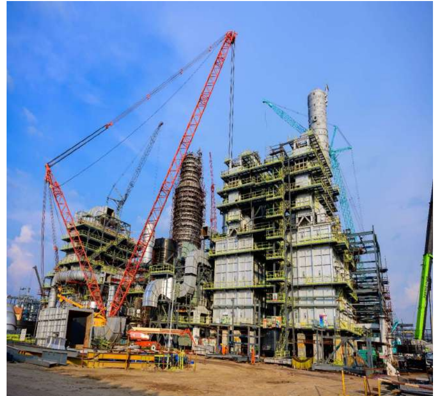
HRRL Project, Rajasthan
