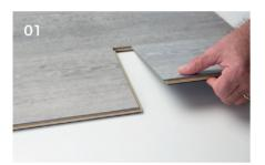
Start by engaging the plank on the long side (angle-system)
