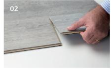
Slide the plank until it reaches the short side of the next plank
