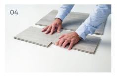
Press with your thumb on both ends of the short side
