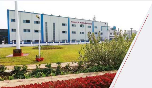
Dadra Paints Plant, Western India
