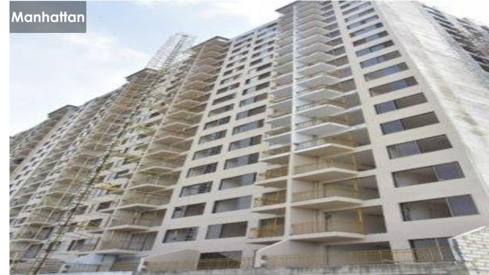
Project Status as on Sept 25
