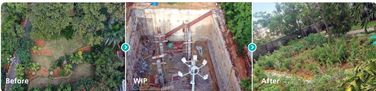
○ Rain water harvesting: 40 lakh litre cistern
