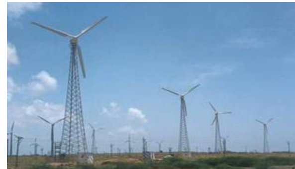
Lamba, Dhank, Pransla - Windmills - 40 wind turbines - 8.6 MW
