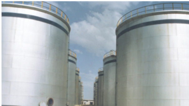
Kandla - Shore tanks - 11 tanks, 13.2 km 3
