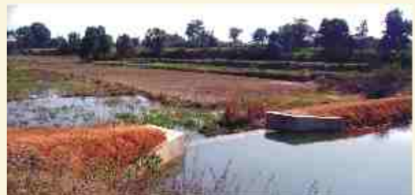
Check dam under KCI's water harvesting programme.
