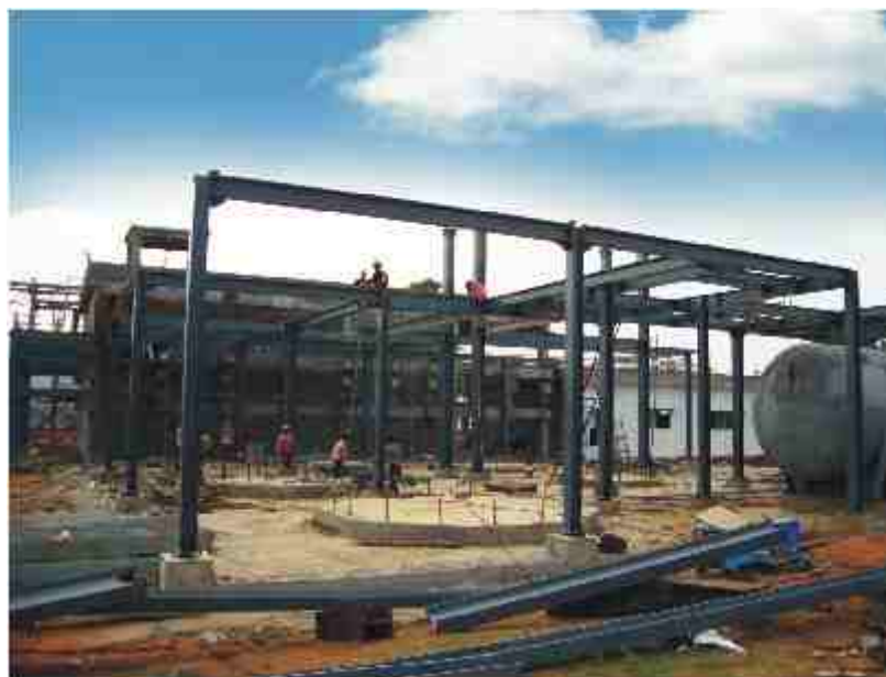
Formaldehyde plant under construction, Vishakhapatnam
