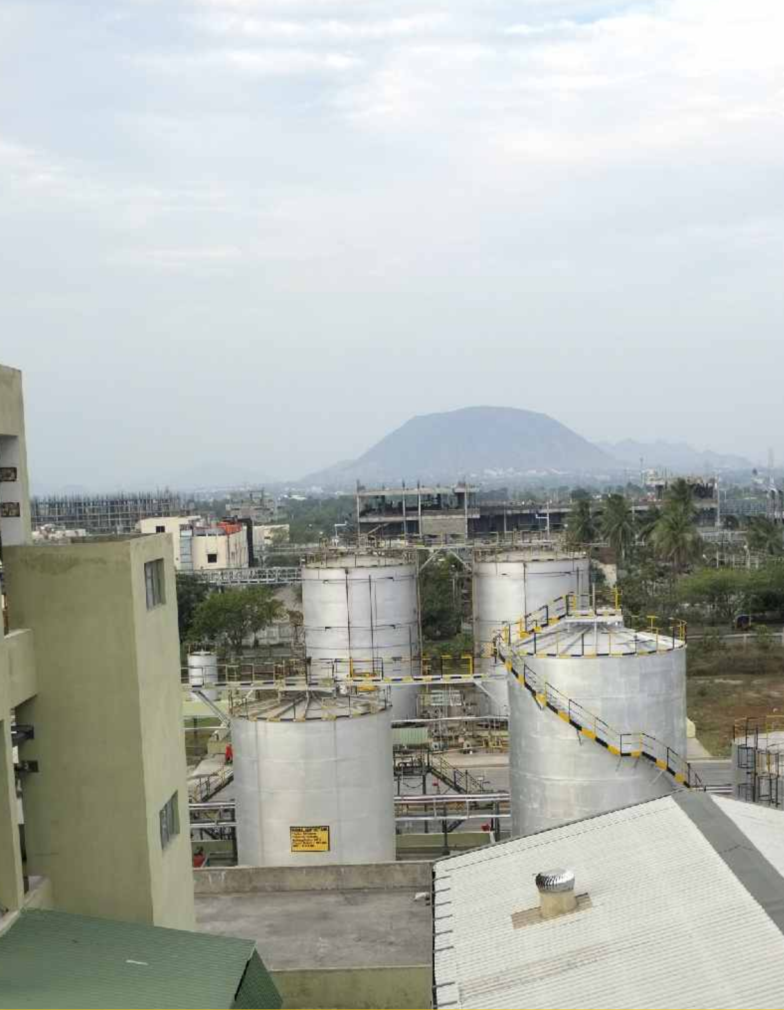
View over the Tank Farm, Vishakhapatnam
