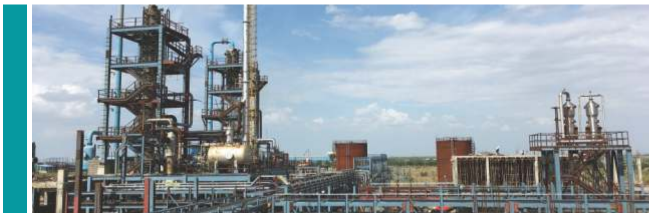
Plant at Naidupeta, Andhra Pradesh
