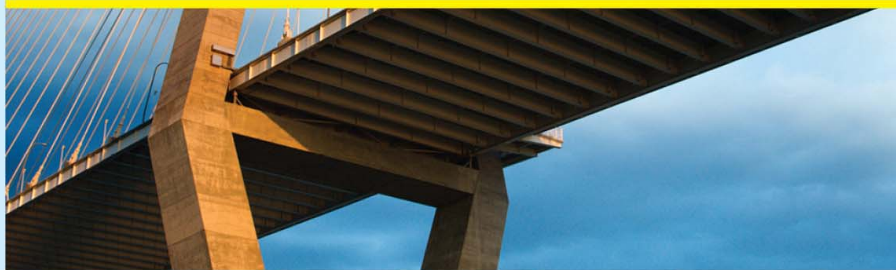
General fabrication and civil construction
