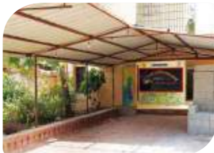
Constructed Classrooms for Primary School in Valsad
