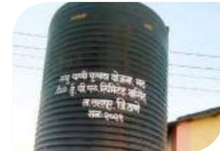
Drinking Water Project in village Madhhal, Vasind, Maharashtra
