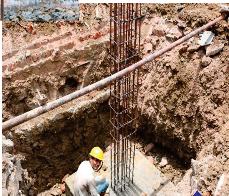
Work in progress for construction of classrooms at Salvad
